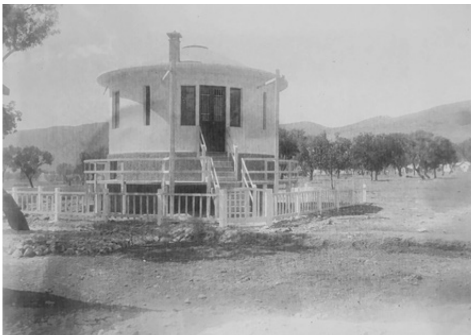
Fig.6.3 Slide portraying one of the asismic huts built by the Brothers Giuseppe and Duilio Torres in Avezzano. (source: Giuseppe Torres, Iuav-Archivio Progetti)
