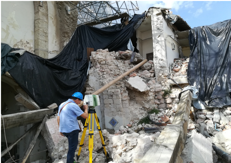
Fig.8.4 Basilica of San Benedetto di Norcia, débris scanning activities (source: authors, October 2019)
