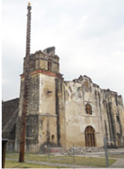
Fig.7.8 Church after the earthquake of 19 September 2017 (source: author)
