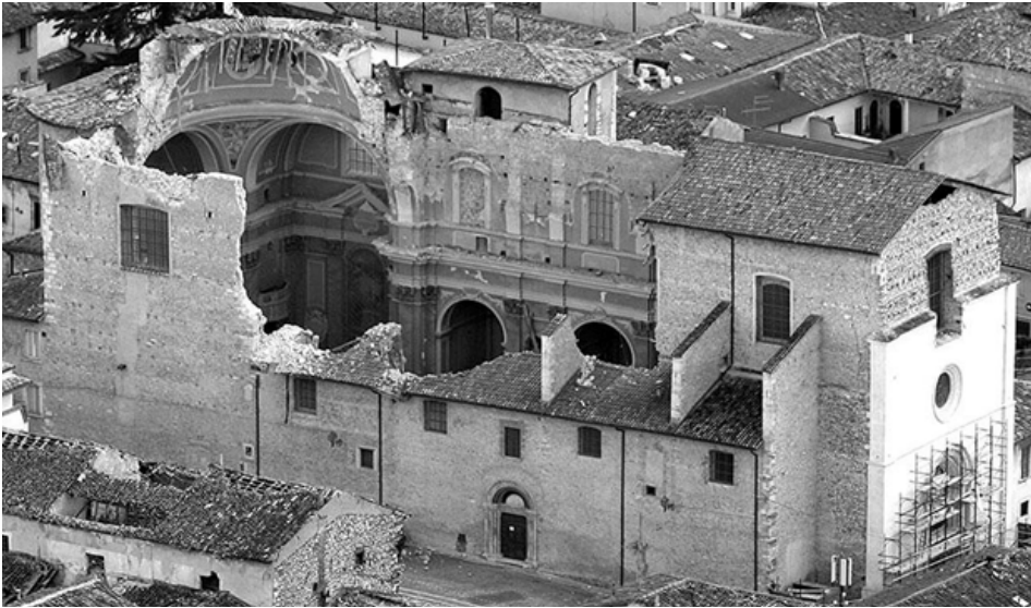
Fig.4.12 St. Maria Paganica Church after 2009 earthquake (source: Civil Protection flight after the earthquake, 2009)
